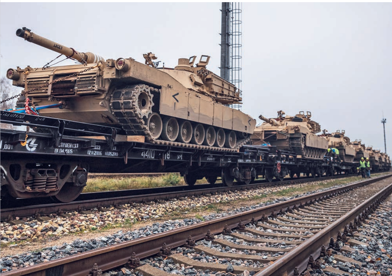
Garkalne railway infrastructure, developed for military needs, opened in 2018. Photo: NBS (National Armed Forces)
